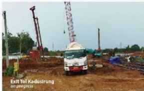
Exit Tol Kadusirung on progress
